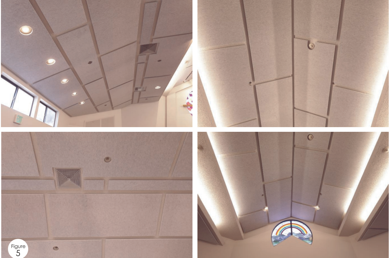
Details of the PolySorb panel layout. Design and installation by Contour Audio & Acoustics.
