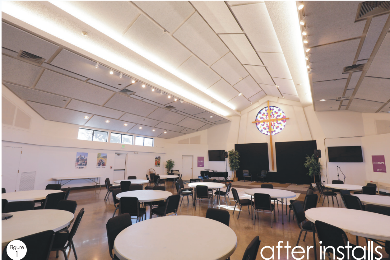
Figure 1 Family Life Center at Abiding Hope Church following installation of PolySorb on the ceiling.
